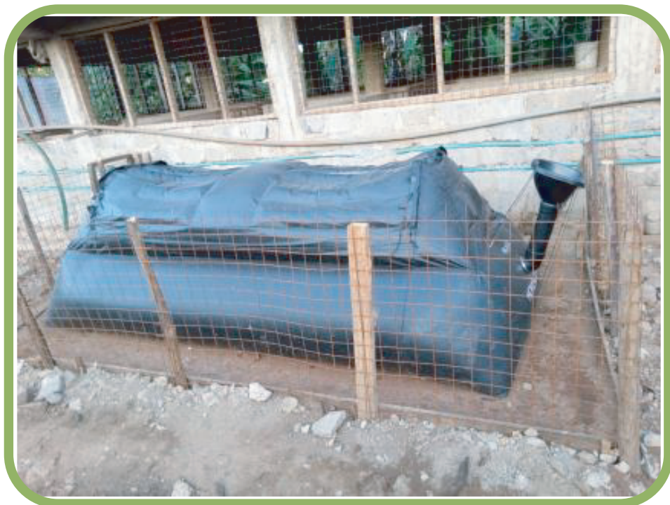
Portable domestic biogas
